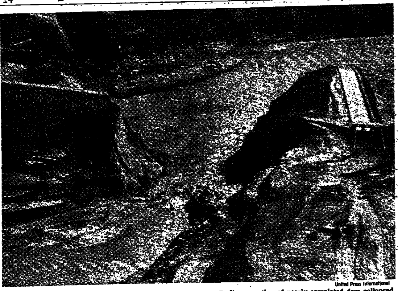
Water rushing through a break in the Teton Dam in Idaho June 5 after a section of nearly completed dam collapsed
